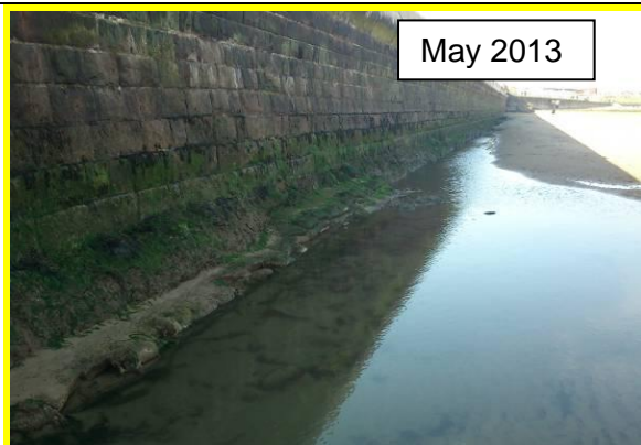
Low beach level in May 2013 exposing seawall toe which is undercut in places and previous concrete bagwork repairs. (Asset Ref. No. 121AB901B0603C03)
