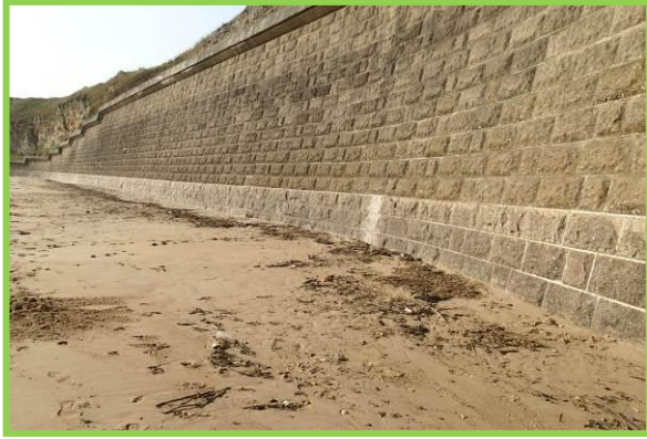
High masonry wall in good overall condition. (Asset Ref. No. 121AB901B0605C01)
