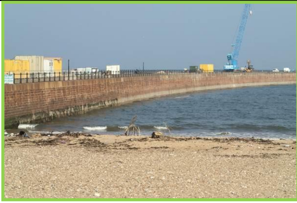
Works underway to refurbish Roker Pier. (Asset Ref. No. 121AB901B0702C04)
