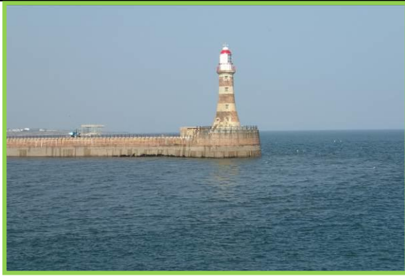
Seaward end of Roker Pier viewed from New South Pier. (Asset Ref. No. 121AB901B0702C04)
