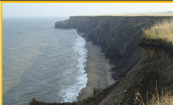
Eroding cliffs at Halliwell Banks. (Partly active) (Asset Ref. No. 121AB901B0804C02)
