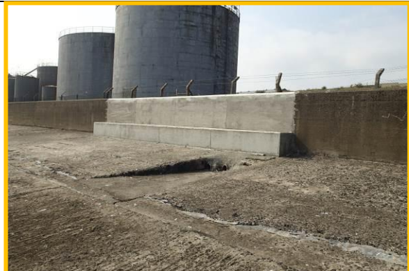
Repaired section of crest wall. (Asset Ref. No. 121AB901B0802C01)
