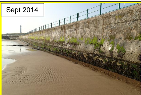
Seawall adjacent to Seaburn Park, showing chloride staining on surface of concrete encasement. Beach levels higher than in May 2013. (Asset Ref. No. 121AB901B0604C01)
