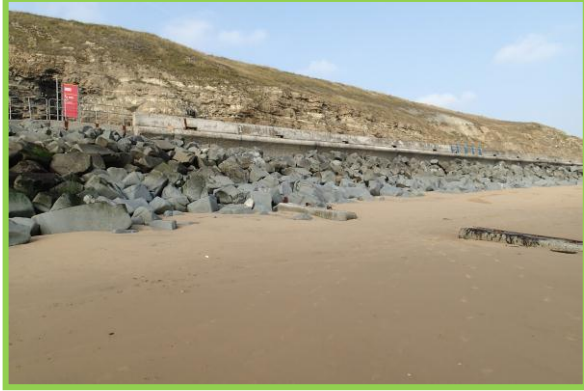
Rock armour in good condition. (Asset Ref. No. 121AB901B0803C02)
