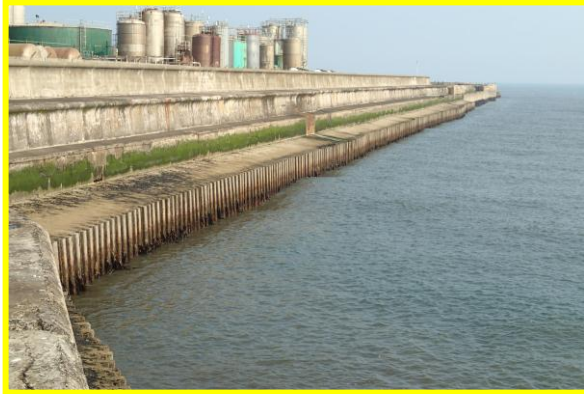
Spur barrier wall. (Asset Ref. No. 121AB901B0802C04)
