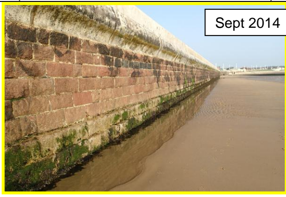
Higher beach level covering toe. Missing mortar / open joints between blocks. (Asset Ref. No. 121AB901B0603C03)
